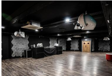
Designed for direct dispersion control, the triangular profile waveguides **ensure an even and predictable acoustic distribution** with a 90° horizontal and 60° vertical pattern. This geometry **reduces unwanted reflections** and concentrates acoustic energy on the audience, being particularly effective in difficult or high-density environments.
